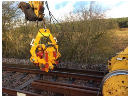
Rail Dragging and Threading
