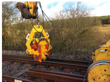
Rail Dragging and Threading
